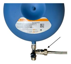
Now mount another water hose (13) on top of the tee (26) onto the other nipple coupling (28).
