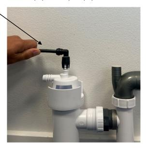
Push the 8 mm push-in elbow (22) into the top of the Siphon (17).
