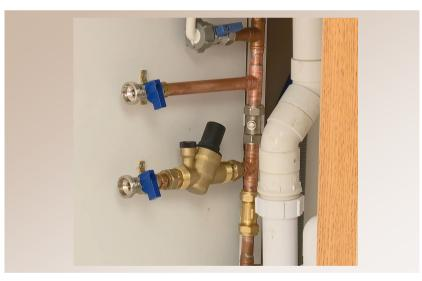
Picture 3: By – Pass set shown in a typical Situation.
